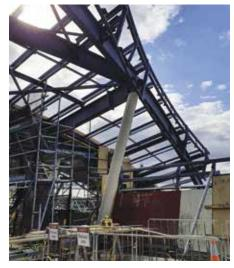
Two examples of the complex connections involve the curved rectangular hollow section beams that help to form the curving glassreinforced concrete façade and the balustrades at the central stairs. To create the curving visual impression, all the secondary steel used to form the central stair balustrade and the façade have varying heights and angles.
