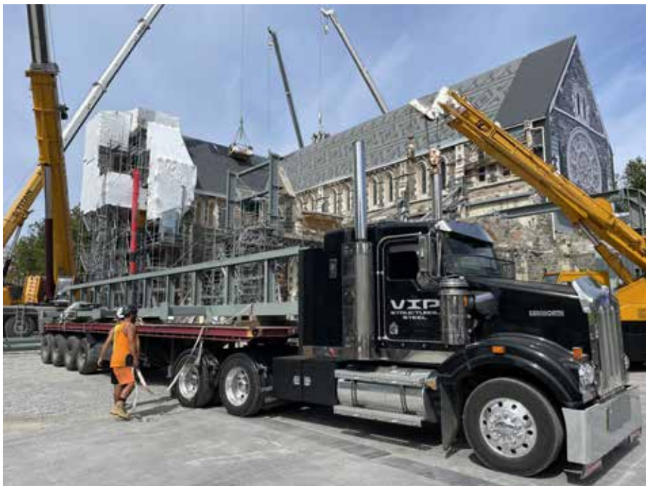
OPPOSITE PAGE AND ABOVE: ONE INNOVATION ON SITE IS THE TEMPORARY SLIDING ROOF OVER THE CROSSING. IT PROTECTS THE HISTORICAL FEATURES WITHIN FROM THE ELEMENTS AND ALLOWS WORKERS SUSPENDED IN A CAGE ON A CRANE TO BE LOWERED THROUGH THE OPENING INTO THE HEART OF THE BUILDING.
