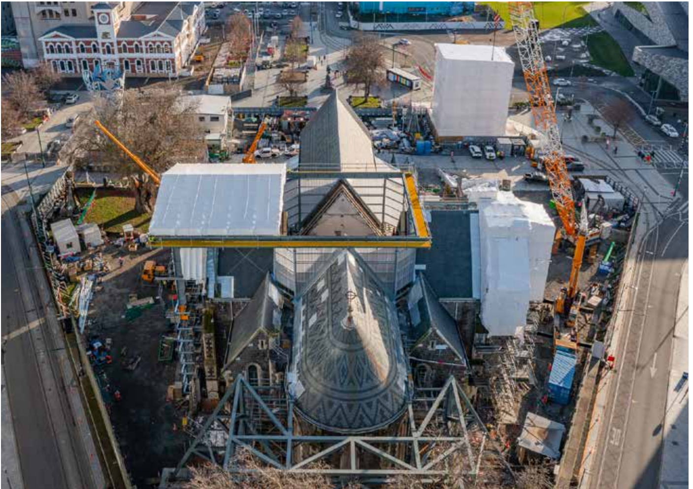
OPPOSITE PAGE AND ABOVE: ONE INNOVATION ON SITE IS THE TEMPORARY SLIDING ROOF OVER THE CROSSING. IT PROTECTS THE HISTORICAL FEATURES WITHIN FROM THE ELEMENTS AND ALLOWS WORKERS SUSPENDED IN A CAGE ON A CRANE TO BE LOWERED THROUGH THE OPENING INTO THE HEART OF THE BUILDING.
