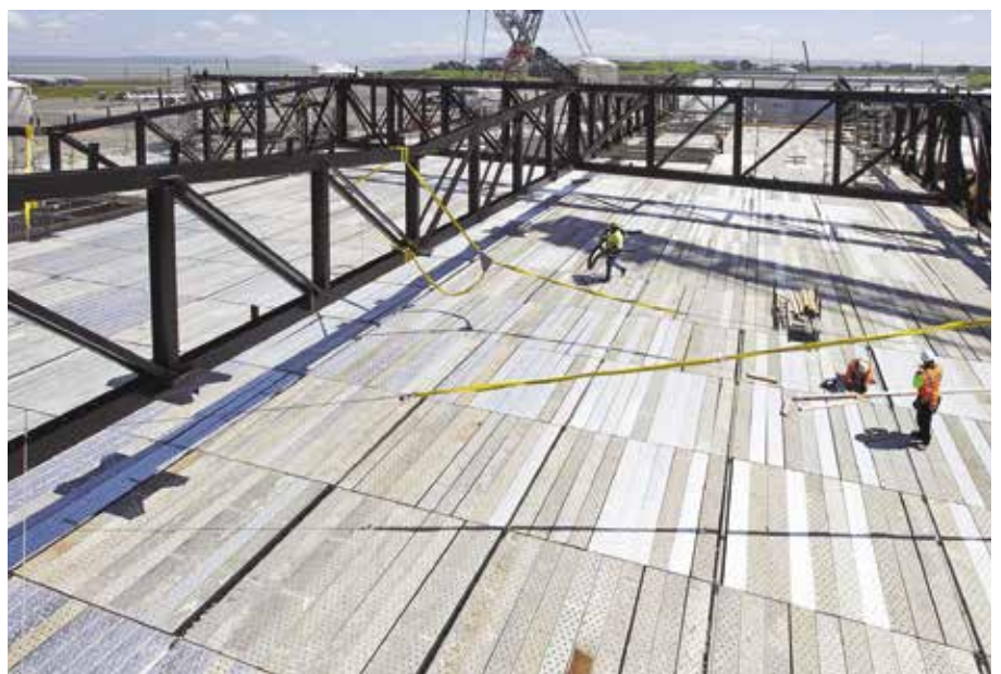
Below: Steel has the ability to deliver wide spans and clear unobstructed space. Auckland International Airport's original 1970's terminal was futureproofed with structural steel, allowing the structure to be repurposed and expanded. The new terminal has double the dwelling space without increasing the overall footprint. (Pictured, Auckland International Airport expansion.)
