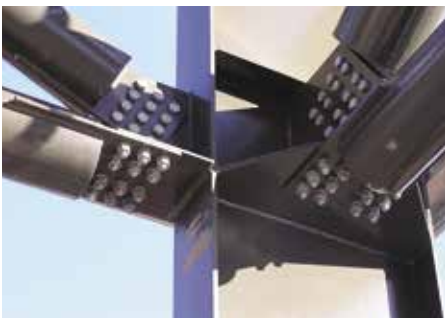
Above: Investment in fabrication technology and workshops, and the modern approach of simple bolted connections, has improved productivity in New Zealand’s structural steel industry.
