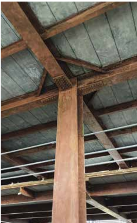
Above: The structural steel elements of The CAB were found to be very sound. Reusing such a large portion of the building vastly reduces its carbon footprint. (Pictured, original 1950's steel in The CAB, Auckland.)
