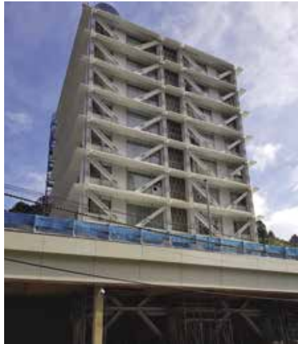
Top Left and right: Another big change in the last 10 years is the advent of retrofitting structures for earthquake strengthening purposes. (Pictured, Chinese Embassy, Wellington.)
