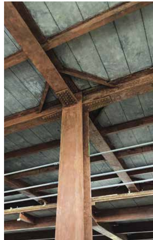
ABOVE: THE STRUCTURAL STEEL ELEMENTS OF THE CAB WERE FOUND TO BE VERY SOUND.
