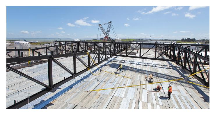
"WORKING WITH STRUCTURAL STEEL IS A HUGE ADVANTAGE IN CONSTRUCTION. NOT ONLY DOES ITS FLEXIBILITY ALLOW US TO COME UP WITH COMPLEX FORMS, BUT ITS LIGHTNESS MEANT THE EXISTING STRUCTURE COULD BE STRENGTHENED WITHOUT ADDITIONAL STRAIN. THIS IS A MASSIVE SUSTAINABILITY WIN AS WE WERE ABLE TO BUILD ON THE ORIGINAL DESIGN INSTEAD OF KNOCKING IT DOWN."
