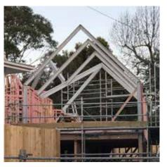
The project boasted a well-coordinated and rapid superstructure installation that saw all of the structural steel for the house erected in just over a day.
