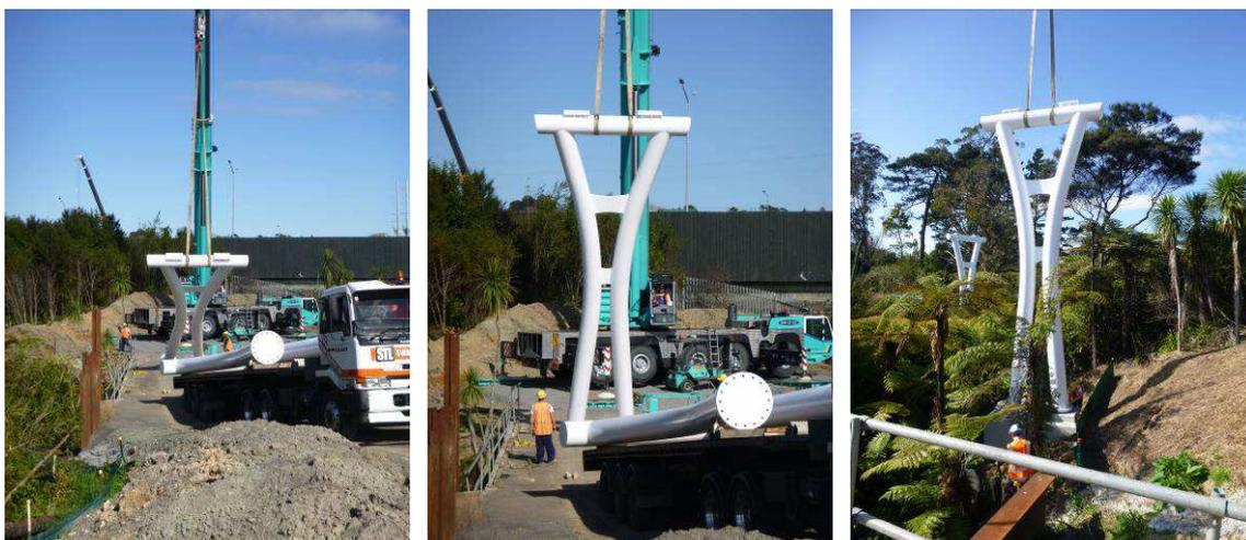
Figure 6. Pier 8 erection.
