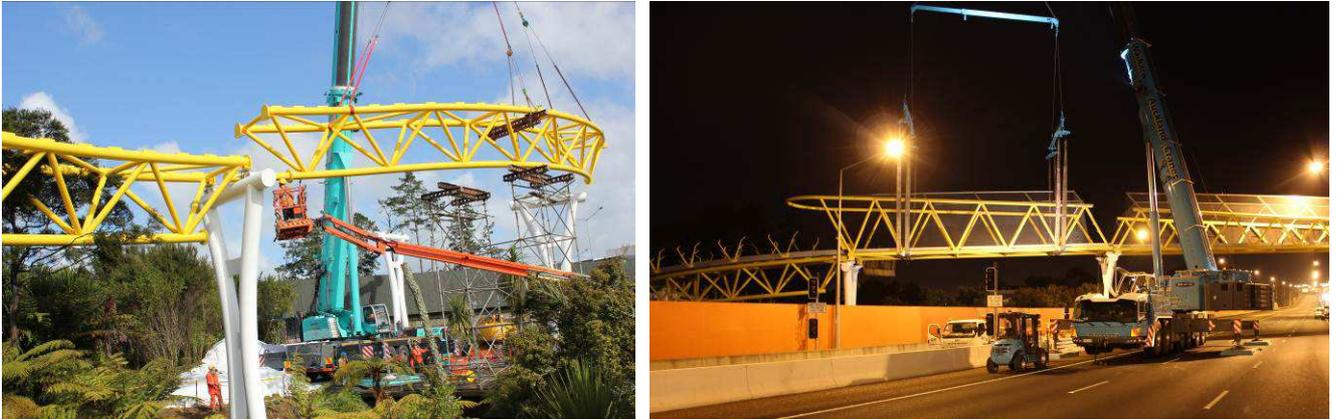
Figure 7. Bridge 2 span 8 lift (left), Span 6 being lifted into place.
