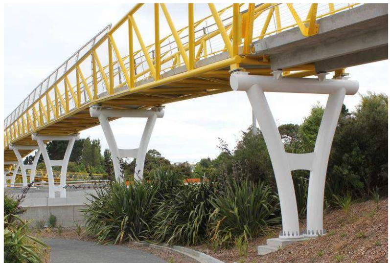
Figure 5. Typical pier arrangement.
