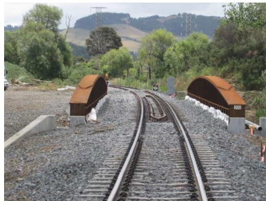
Bridges 299 and 300 NIMT – Two single track decks (36m span)
