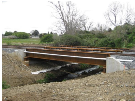
Bridge 312 NIMT – Two single track decks side by side (14m span)
