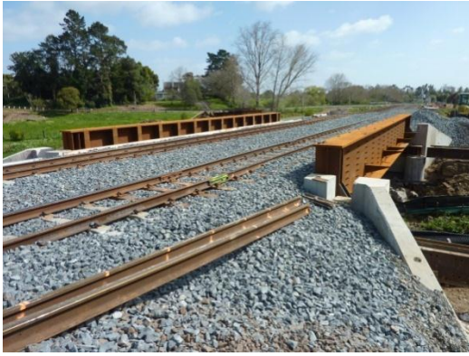
Bridge 332 NIMT – Twin track on a single deck (17m span)
