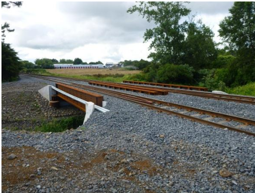
Bridge 312 NIMT – Two single track decks side by side (14m span)
