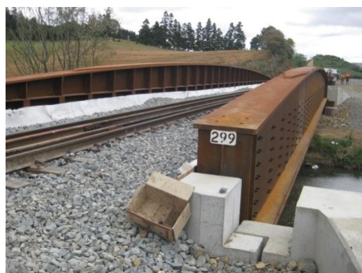
Bridges 299 and 300 NIMT – Two single track decks (36m span)
