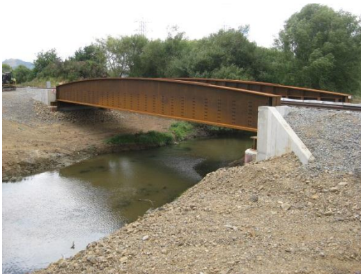
Bridges 299 and 300 NIMT – Two single track decks (36m span)
