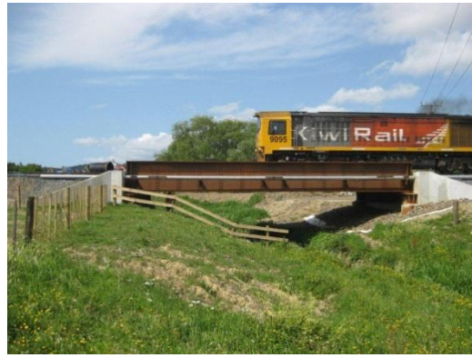
Bridge 332 NIMT – Twin track on a single deck (17m span)
