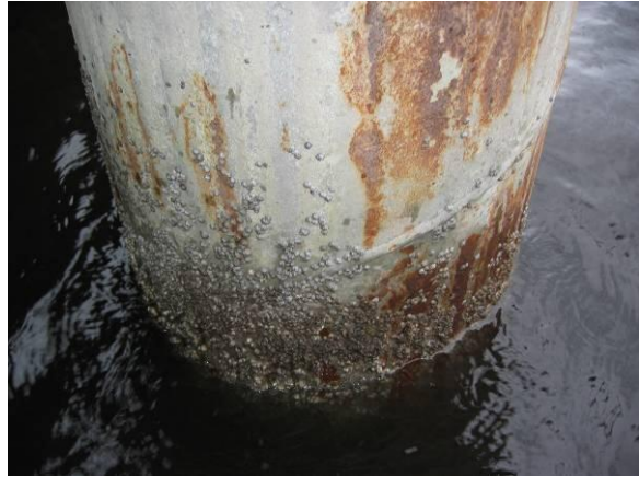
Figure 12. TSA "failure" on pile
