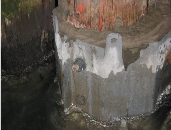
Figure 11. TSA on pile jacket
