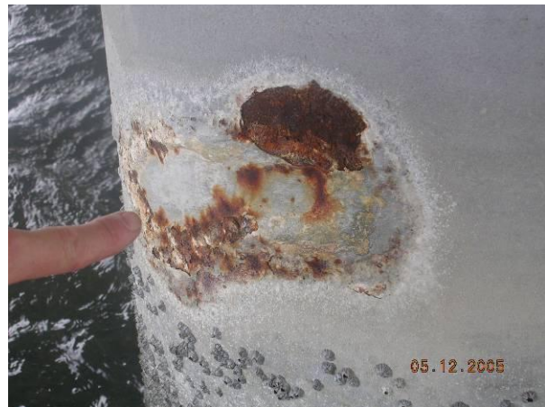
Figure 14. Failure of TSA repair?
