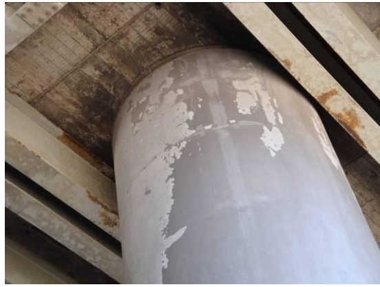
Figure 16. Seal coat delaminating off TSZ
