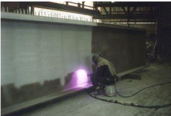
Figure 3. Arc spraying Orewa Bridge Beam
