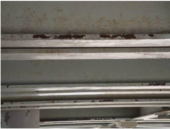
Figure 15. Duplex TSZ failure on a TOB catch frame
