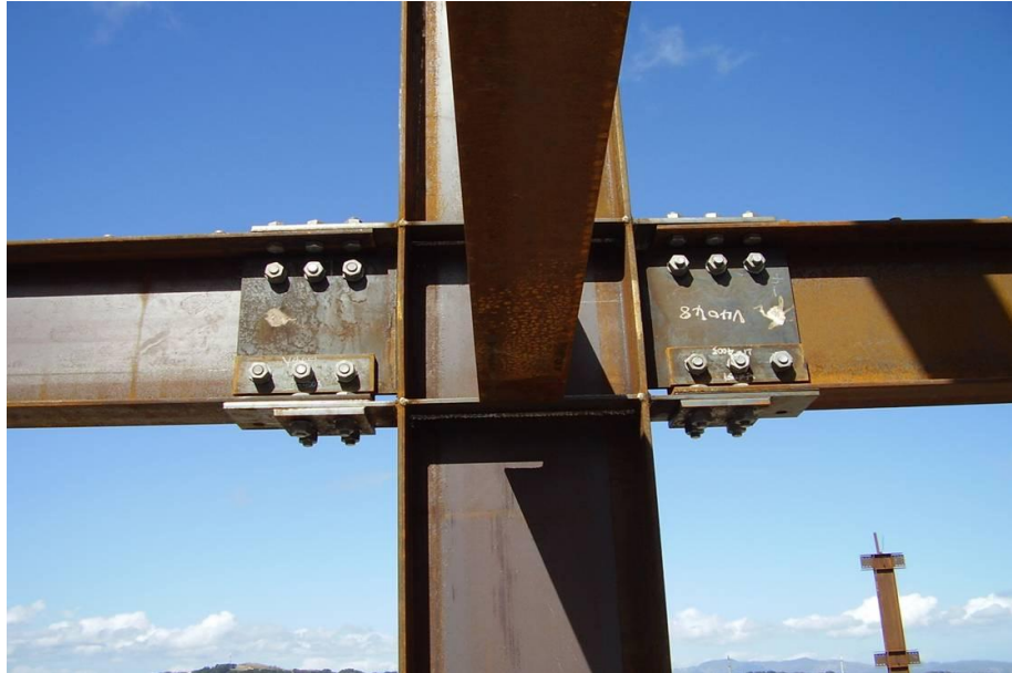
Figure 6: Sliding hinge joint and beam column – Te Puni Student Village
