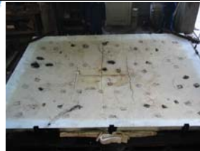
D147 top surface crack pattern
