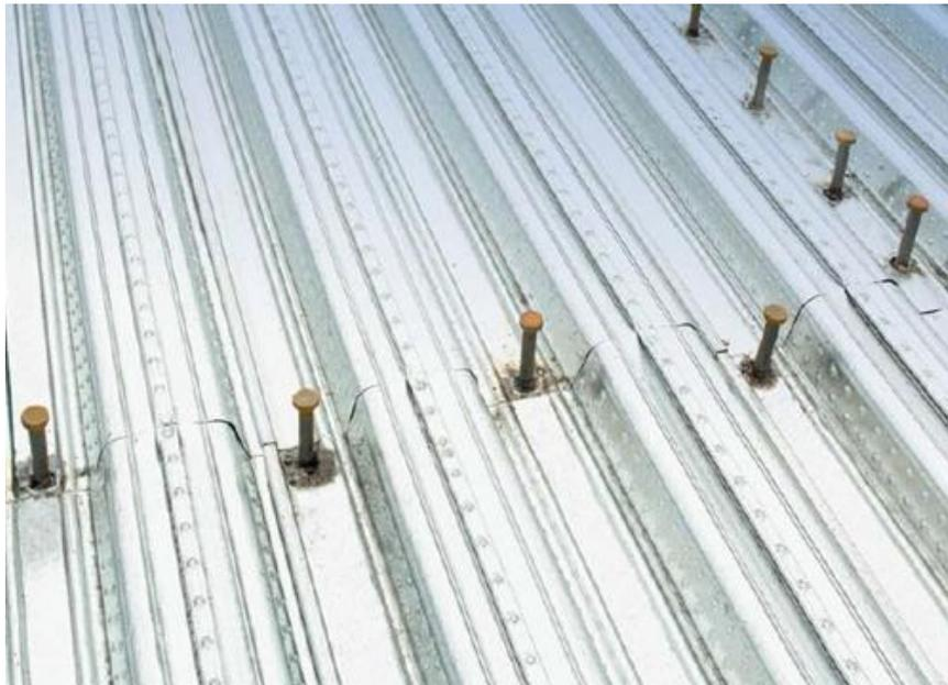
Figure 5. Butt joint in decking (correct positioning of single stud per trough)
