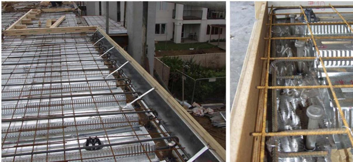
Figure 7: Slab edge form at spandrel beam (Clifton, El Sarraf, 2005)
