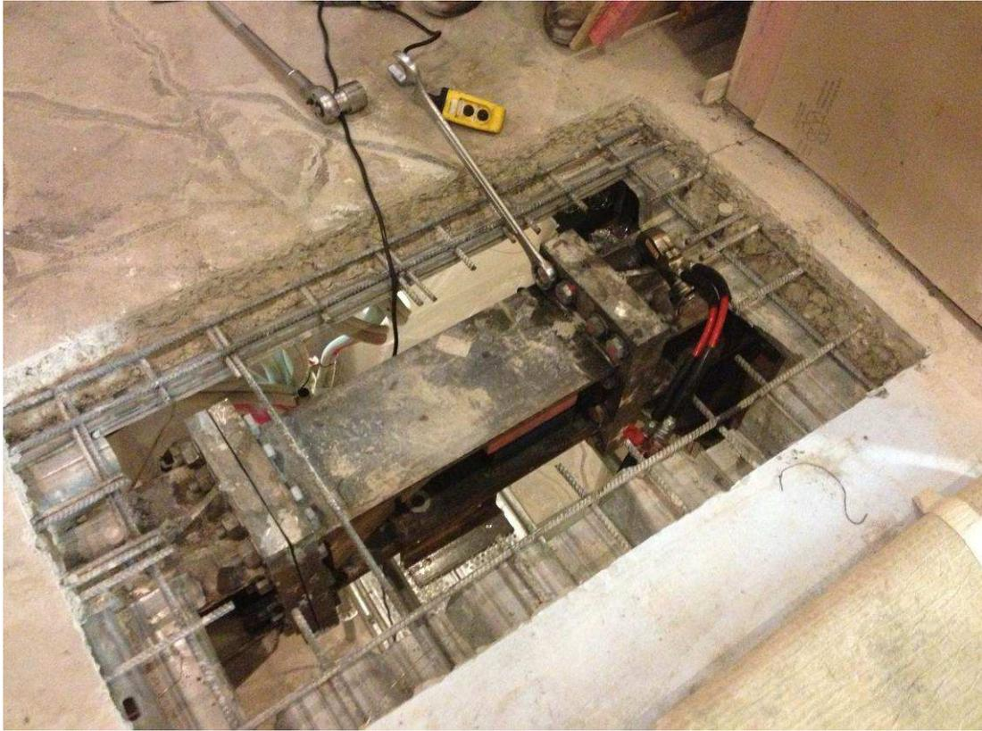
Figure 11: Bolted-in active link during bolt tensioning. Image Spiire New Zealand Ltd.
