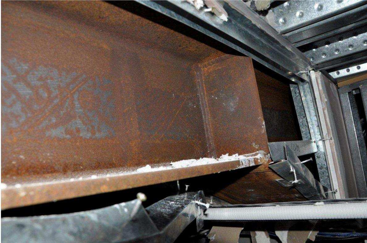
Figure 1: Active link with diagonal Luders lines. Image Spiire New Zealand Ltd.
