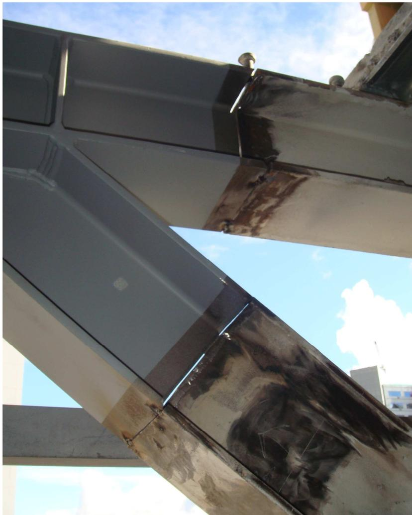
Figure 7: Active link replacement location prior to welding. Image courtesy of Fortis Construction.
