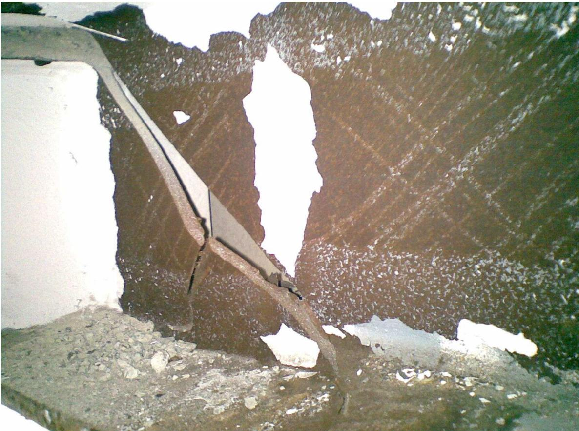
Figure 3: Fractured active link. Image Spiire New Zealand Ltd.
