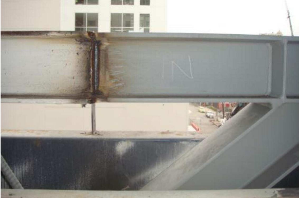
Figure 8: Replaced active link welded in place. Image courtesy of Fortis Construction.
