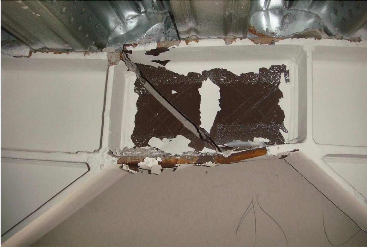
Figure 2: Fractured active link. Image Spiire New Zealand Ltd.
