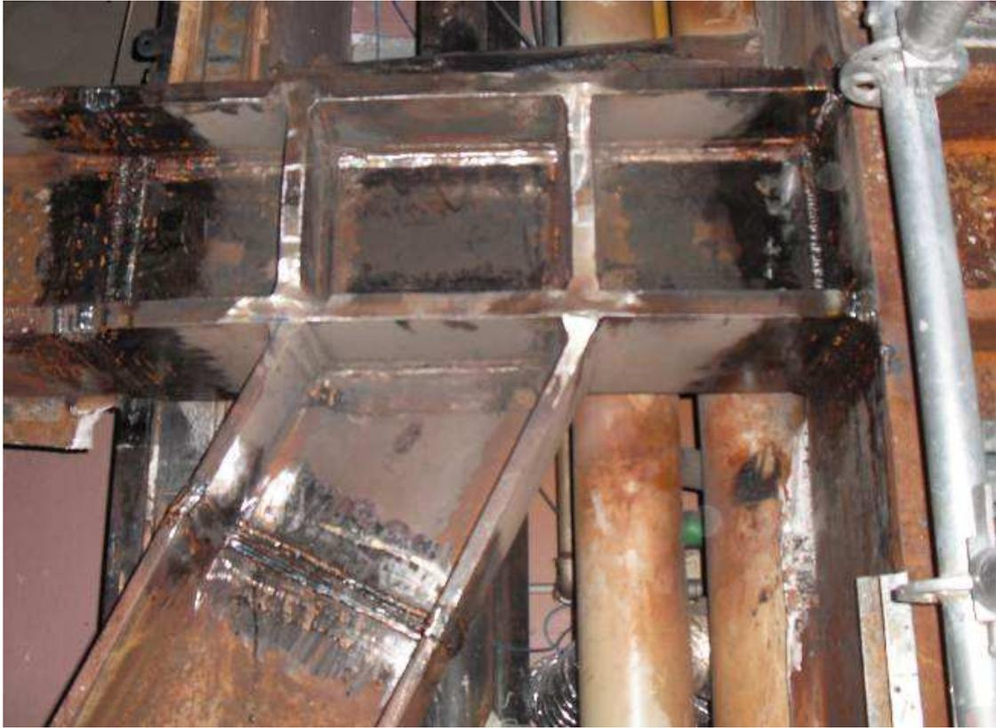
Figure 12: Welded-in active link. Image courtesy of Fortis Construction.
