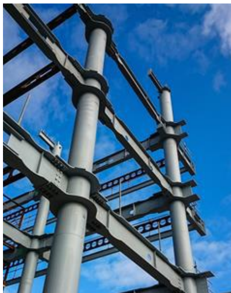
Figure 4. Two way moment resisting system adopted for the Christchurch Justice and Emergency Services Precinct project
