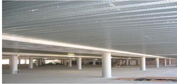
Figure 1. Soffit of a one-way composite slab and beam floor system.
