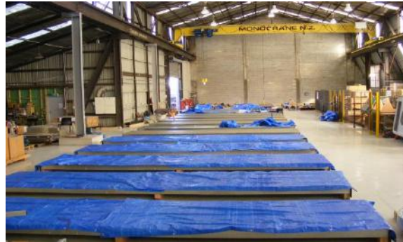
Figure 1. Composite Slabs after Concrete Casting.
