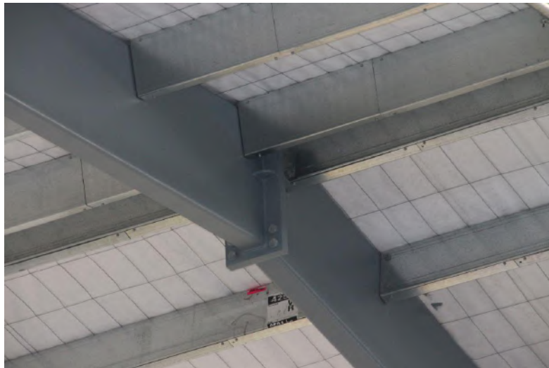
Figure 4. A typical example of the vermin proof NTBB design, combined with the inclusion of nested purlins.
