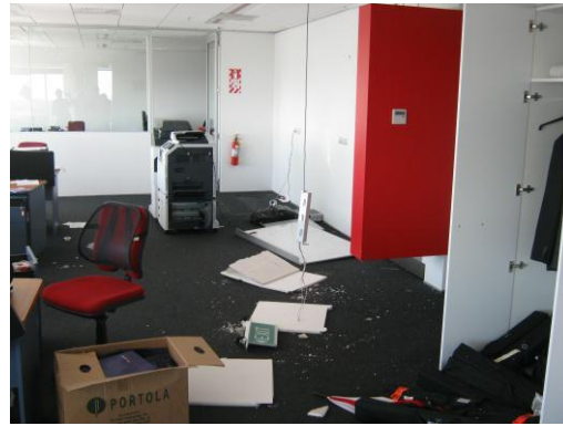
(d) Typical office following 22 Feb 2011 earthquake [C Clifton]
