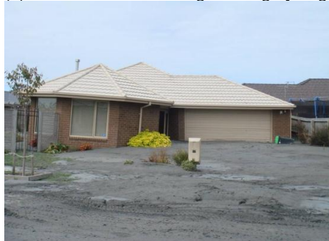
(c) Ground instability [M Pender]
