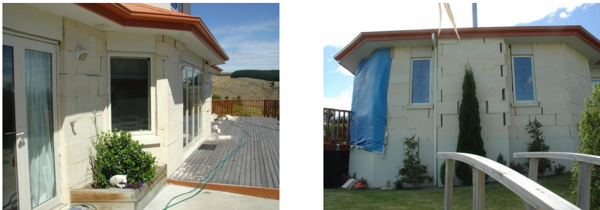
Figure 7 Two storey light steel frame house with Oamaru stone cladding [T Just]
