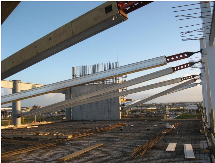
Figure 8: As erection takes place, a series of diagonal props back to the interior side of the building is needed to maintain the stability of the steelwork while it undergoes deflections.
