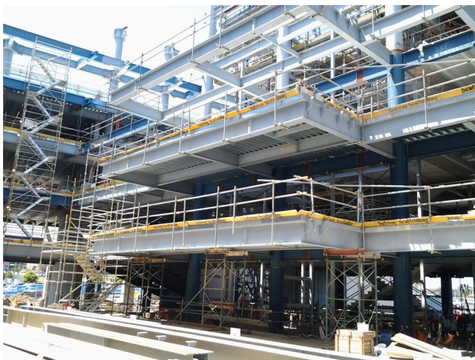
Figure 10. The bridges (to the left) will be suspended from large atrium roof trusses, as will the cantilevered lift lobbies (centre).
