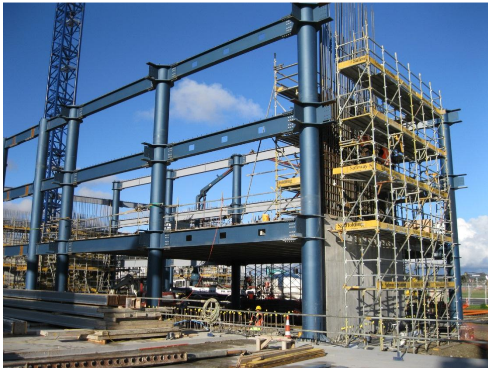
Figure 5. The interior sides of the building have conventional column and beam steel frames, utilising concrete-filled Circular Hollow Sections (CHSs) and a collar arrangement for the beam to column connections. The CHSs were fabricated by Jensen Steel Fabricators of Tauranga
