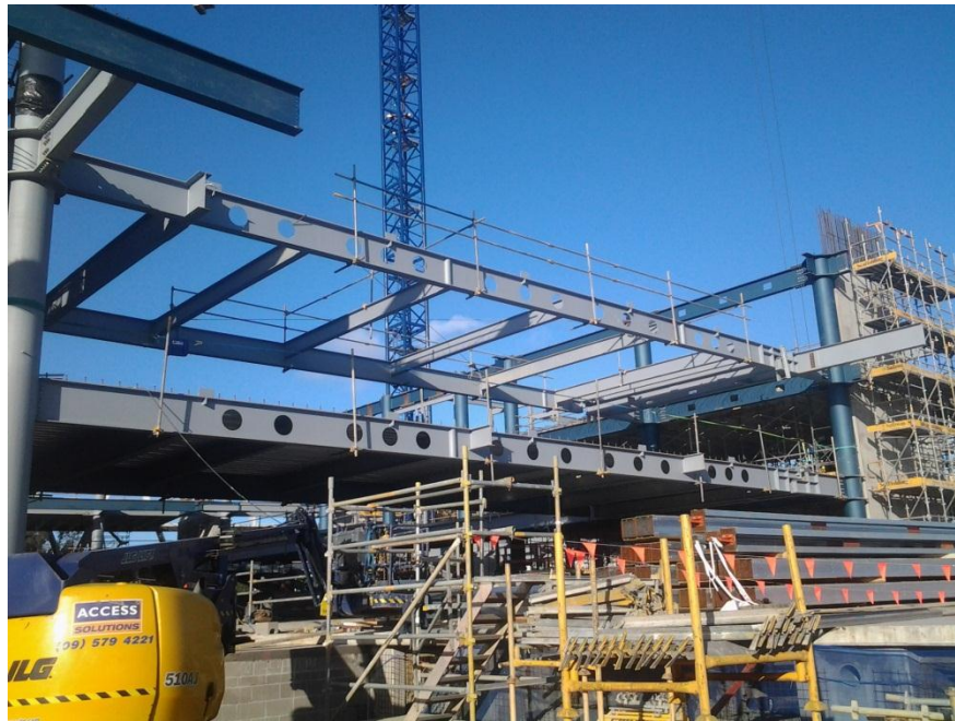
Figure 9. The first two of six 25m-long bridges connect the north and south elements of the building at the western end of the atrium.
