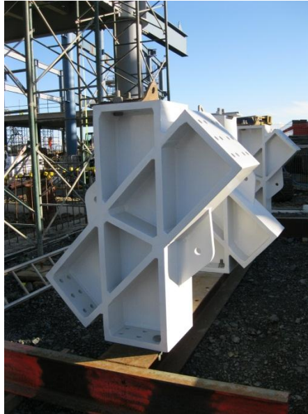
Figure 4. One of the 15 “X” nodes, a centre-point of the diagrid. D&H Steel also fabricated 18 “Y” nodes for the bottom points and 16 “V” nodes for the top points.
