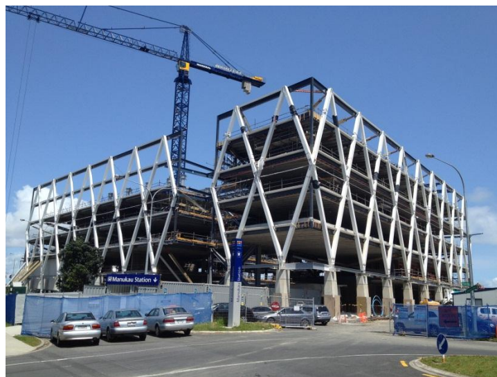
Figure 3. Construction of the diagrid, which extends five levels to roof height.
