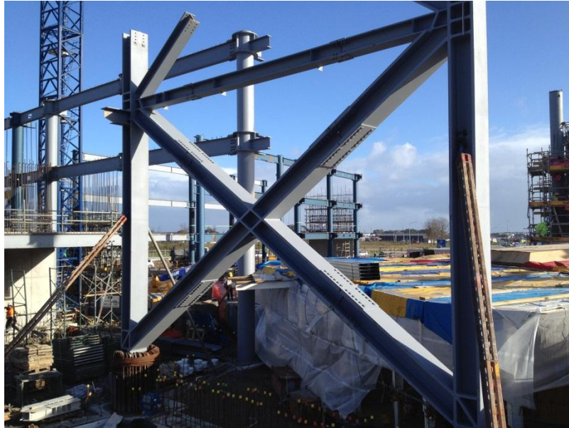
Figure 6. A crucial Eccentrically Braced Frame, this was fabricated for MJH Engineering by D&H Steel from 60mm flange plates with a 50mm web using full penetration welds.
