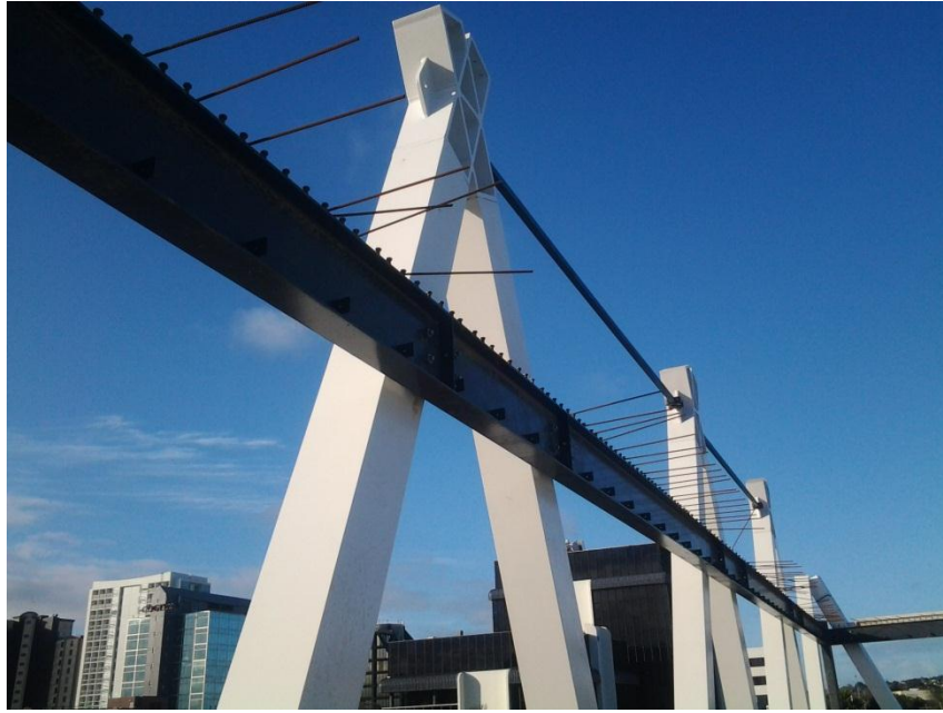
Figure 7. The beam to support the flooring system is located inside the line of the raking frame, resulting in an out-of-plane torque.
