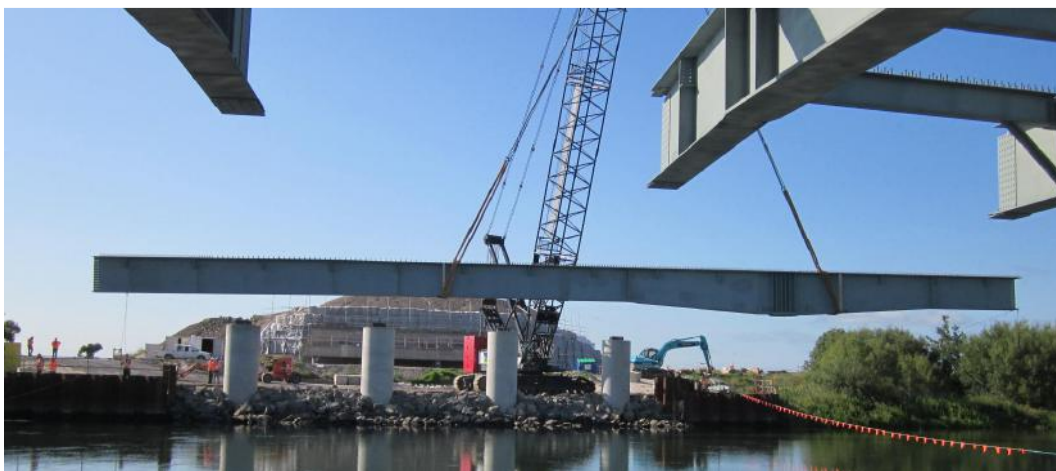
Figure 6. Lifting of main girder sections – 60m long spliced section.
