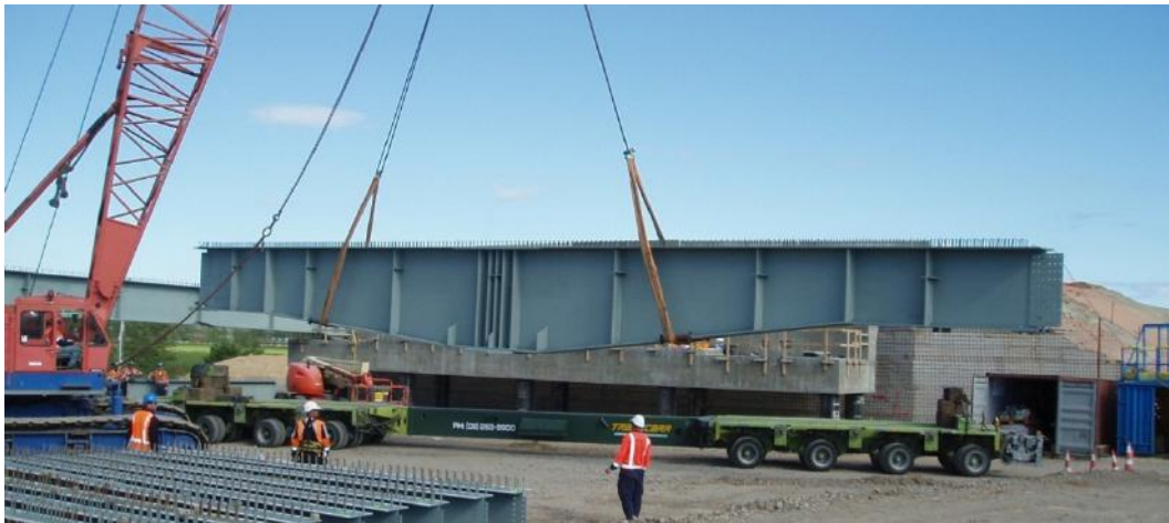
Figure 5. Lifting of main girder sections – 30m section.
