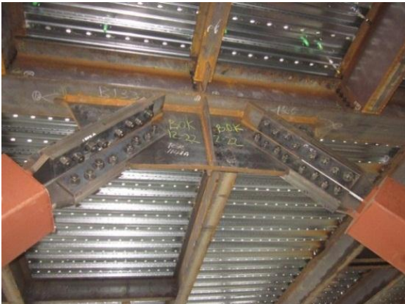
Figure 10 (left) Example of Bolted Splice Connection (Image provided courtesy of Seismic Isolation Engineering, Inc.) and Figure 11 (right) Example of Pinned Connection.
