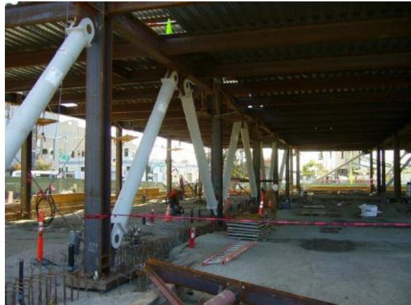
Figure 10 (left) Example of Bolted Splice Connection (Image provided courtesy of Seismic Isolation Engineering, Inc.) and Figure 11 (right) Example of Pinned Connection.
