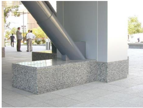
Figure 5. Unbonded Brace™ connection in an exterior exposed application
