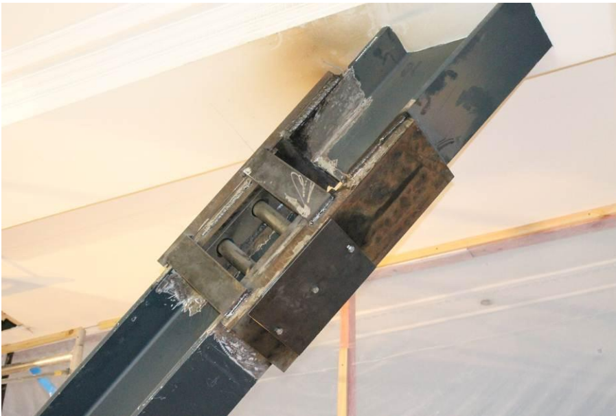
Figure 9. Insitu completed damper.
