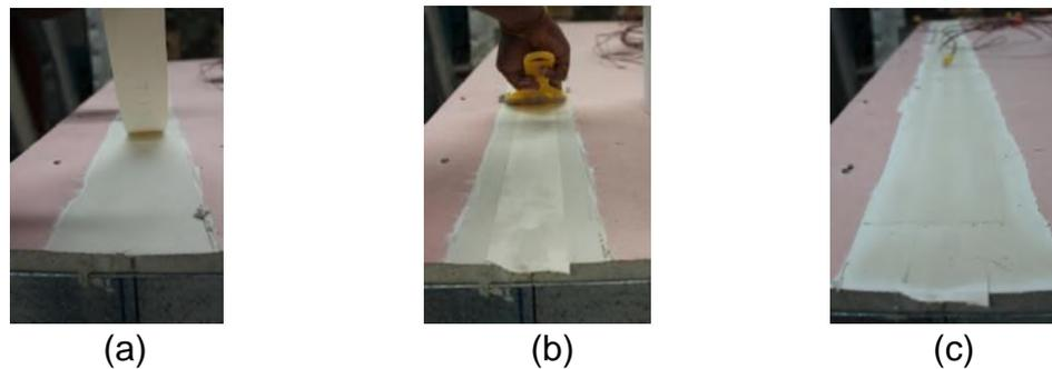
Figure 3. Plasterboard lining and joint sealing
