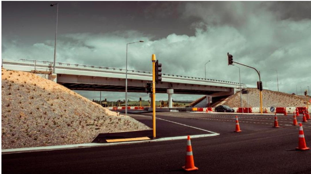
Figure 10 Bridge at completion
