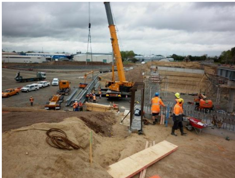
Figure 8 Photos of steelwork erection
