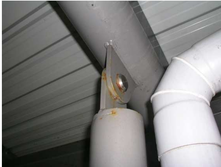
Figure 4: Bimetallic Corrosion
