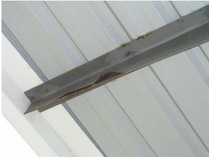
Figure 2: Coating Delamination
