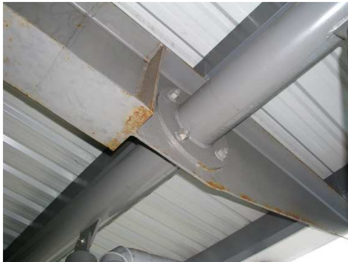
Figure 1: Exposed Girder and CHS
