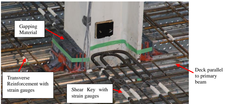
Figure 4: Shear Key Construction Details around Column
