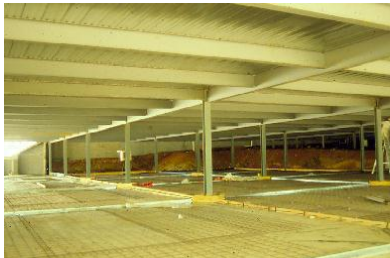
Figure 8. Composite Steel-Concrete Beam and Slab System, Australia
