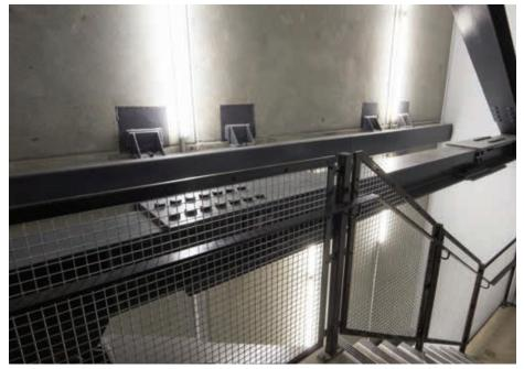
Designed after the Christchurch earthquakes, Te Piringa's seismic preparedness was considered – and it's impressive. Even when exposed to large earthquakes, the steel absorbs seismic forces beam to beam due to their rotation capacity. This system is an alternative in New Zealand and a proprietary product, with just a few global suppliers. "THE TOWER'S STRUCTURE AND MONOLITHIC APPEARANCE EXUDE STRENGTH AND RIGIDITY. TE PIRINGA PAYS TRIBUTE TO LAW, WHICH IS A CORNERSTONE OF ANY CIVILISED SOCIETY."
