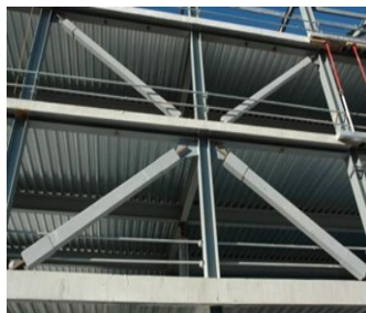
Buckling Restrained Braced Frame (BRBF)
