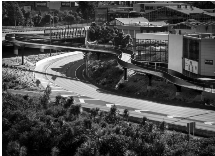
Excellence in Steel Awards 2017 Supreme Overall Winner: Canada Street Bridge, PFS Engineering
